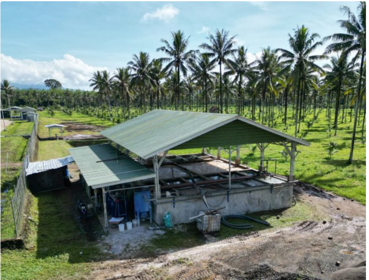
Dewacoco Waste Water Treatment Plant (WWTP)
